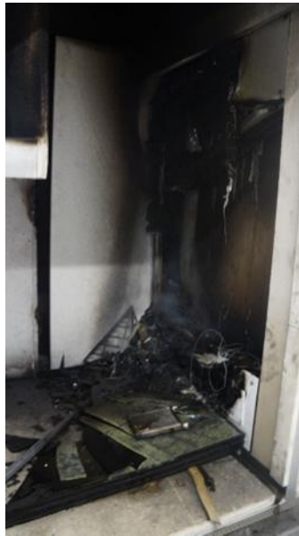
FIGURE 46: SMART WINDOW AFTER THE END OF THE TEST.
