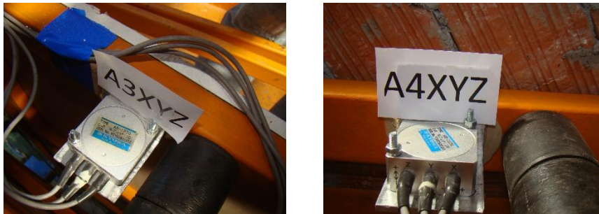
FIGURE 108: INSTRUMENTATION SET-UP: ACCELEROMETERS PLACED AT MEASUREMENT POINTS A3 AND A4 (SMARTWALL)
