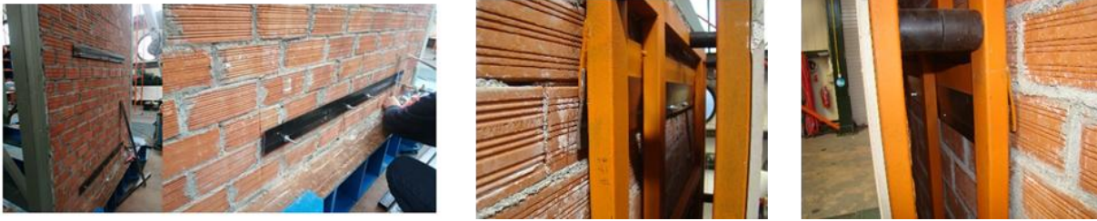
FIGURE 17: FIXING SMARTWALL TO BRICK WALL- Z CLIPS.
