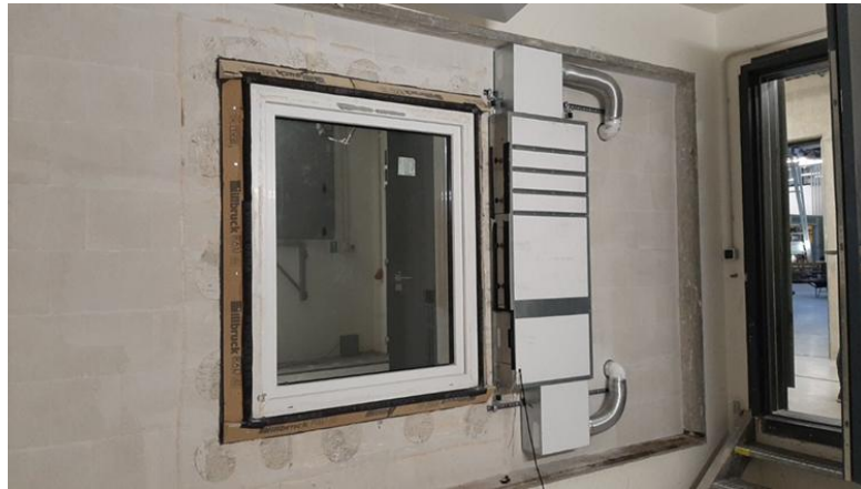
FIGURE 49: eAHC UNIT INSTALLATION DURING THE FULL-SCALE MODEL MEASUREMENT.
