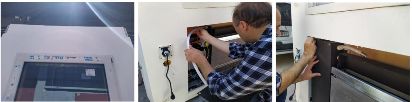
FIGURE 5: (LEFT): WINDOW'S WATER SPLASH TEST, (MIDDLE): ACTIVE FIRE PROTECTION SYSTEM TEST, (RIGHT): TOOLBOX CHECK
