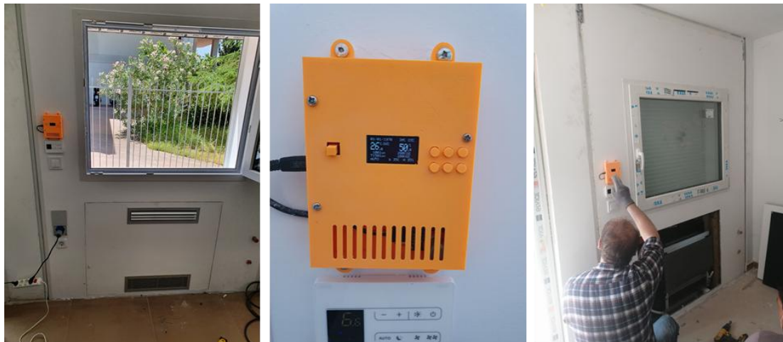
FIGURE 8: (LEFT) FAN-COIL AIR BLOW TEST, (MIDDLE): AMSCOPE TESTING, (RIGHT) AMSCOPE PROGRAMMING.
