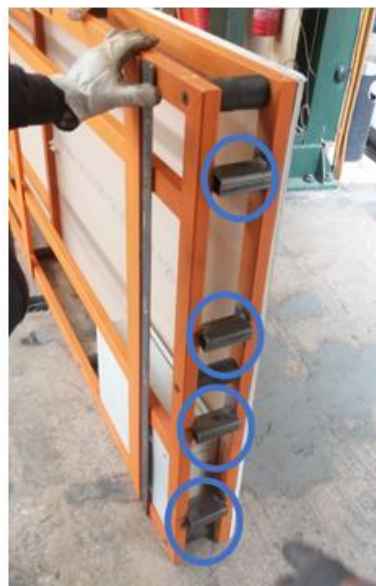
FIGURE 106: FIXING SMARTWALL TO BRICK WALL- BASE SUPPORTS.
