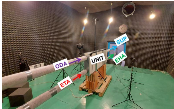
FIGURE 47: NOISE MEASUREMENT IN THE ANECHOIC ACOUSTIC LABORATORY – NOISE FROM THE AIR HANDLING UNIT BODY. SUP – SUPPLY OF AIR TO THE ROOM; ETA – EXTRACTION OF AIR FROM THE ROOM; EHA – EXHAUST AIR OUTLET TO THE OUTDOOR ENVIRONMENT, ODA – OUTDOOR AIR INLET
