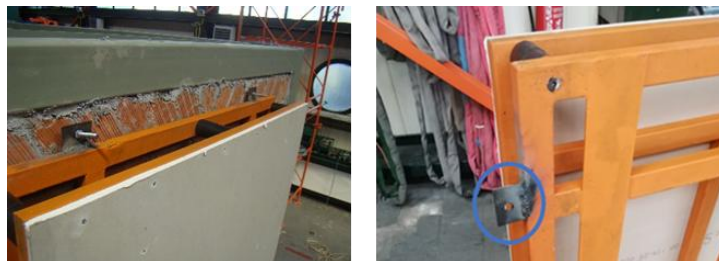
FIGURE 16: FIXING SMARTWALL TO BRICK WALL- TOP ANCHORS.
