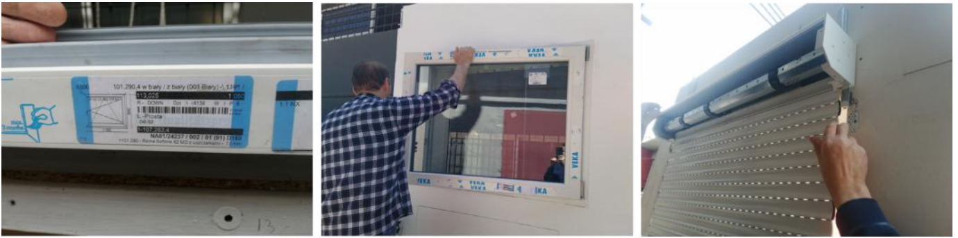
FIGURE 4: (LEFT): WINDOW'S TYPE CHECK, (MIDDLE): WINDOW TILTING AND HINGES TEST, (RIGHT): ROLLER BLINDS STRAP RE-TENSIONING.
