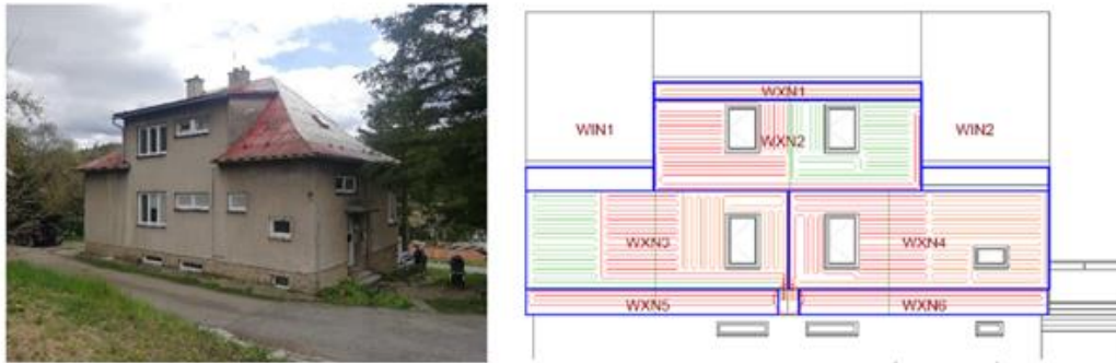
FIGURE 1.3: DEMONSTRATION BUILDING IN KASAVA AT THE PRE-RENOVATION STATE (LEFT) AND A SCHEMATIC OF THE PANELS OF THE NORTH FAÇADE OF THE BUILDING SHOWING THE HEATING MEANDERS (WATER PIPING)
