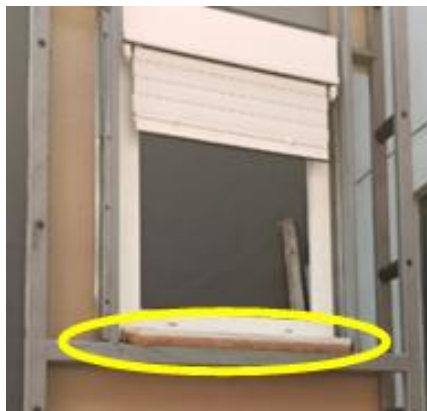
FIGURE 60: CORK SHEET INSTALLED BETWEEN THE WINDOW FRAME AND THE SILL
